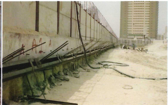
464 tie-back anchors stressing work done successfully at Mixed murur site in Ajman.
