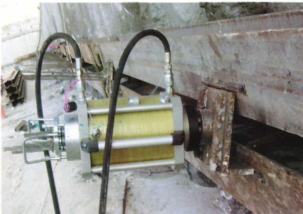
464 tie-back anchors stressing work done successfully at Mixed murur site in Ajman.
